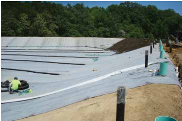
Figure 3-1. Installation of BENTOMAT CL in a typical wastewater lagoon. Inlet pipes in foreground.
